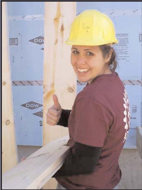
Amanda Reibel, president of the UMF Rotaract Club, gave thumbs up to her experience with the university community service group on the Auburn Habitat for Humanity construction site. (UMF photo)
